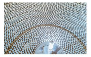
SunMax Premium Reflect Thick is a high reflectivity flat solar mirror available in thickness 3 mm and 4 mm. SunMax Premium Reflect Thick is perfectly suited for use in power tower and linear Fresnel reflectors. SunMax Premium Reflect is designed to provide customers with the highest possible reflectivity and the required durability thanks to its composition. SunMax Premium Reflect conforms to EN1036.
